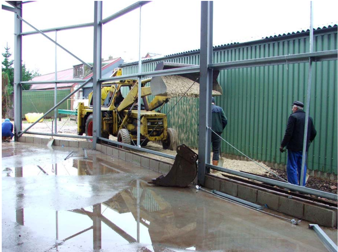
Stoning up the siding 7 prior to the cladding
