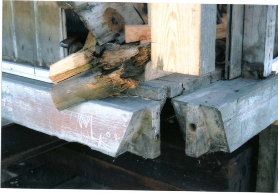
Jointing detail of leg number three, note the excellent condition of the tenons
