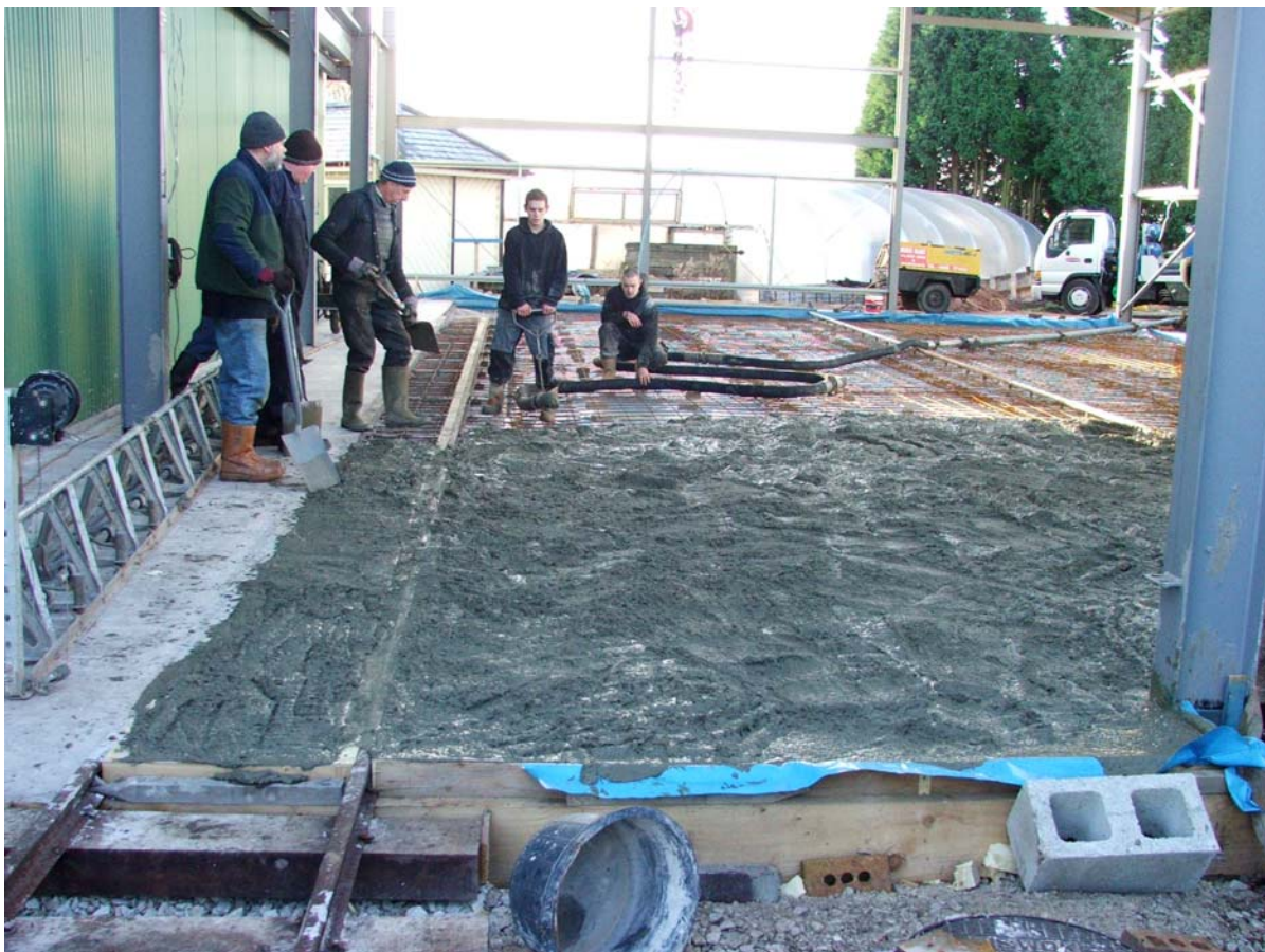
The second pour well underway, with the first load almost discharged
