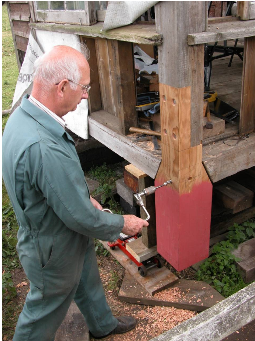
Roger drilling the new corner leg for the tie bolts, note the half joint and below the spliced joint on one of the boards Ray Ashdown
