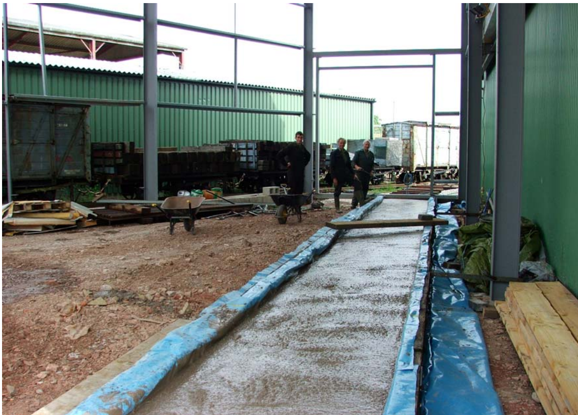
The second concrete gang laying the foundation for the workshop track
