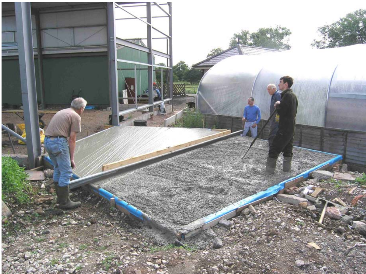
The concrete gang, tamping the pad at the rear of the workshop.
