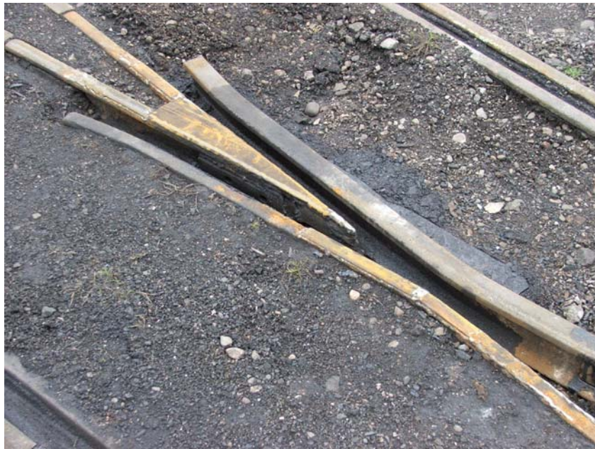
The newly fabricated crossing vee on the old Leighton point on the pit road
